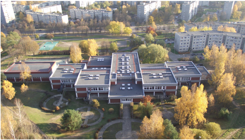
Figure 6. School segments with direct accesses to a yard were joined by the communication corridors arranged breadthwise and lengthwise the slope. View from above. Secondary School for 1284 students in Lazdynai District, Vilnius, 1972–74, architect Česlovas Mazūras [photo by Liutauras Nekrošius].
