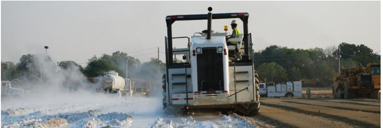
Fig 27. Binder spreading works performed with a special machine
