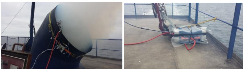
Fig. 21. TESTO 350 measuring device in the scrubber exhaust gas pipe
