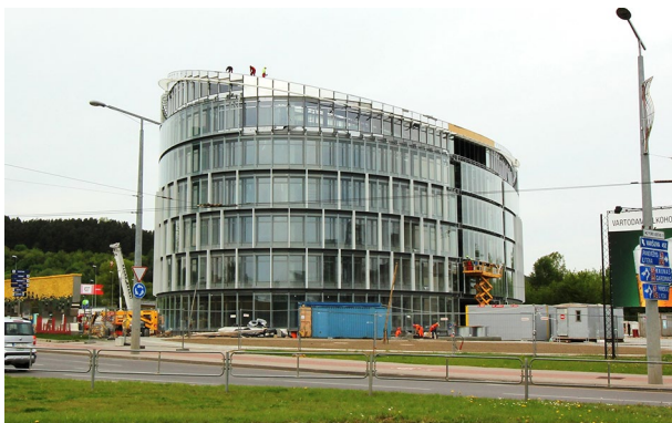
Fig. 1. An original office building, Vilnius
