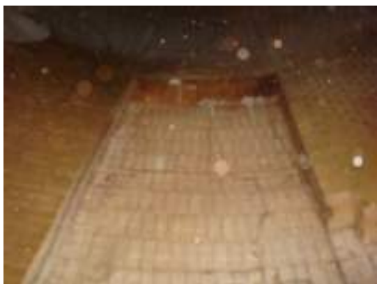
Fig. 2: Panels unlocked due to cracked telescopic bricks at the tongue
