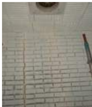
Fig. 2: Deteriorated refractory wall.
