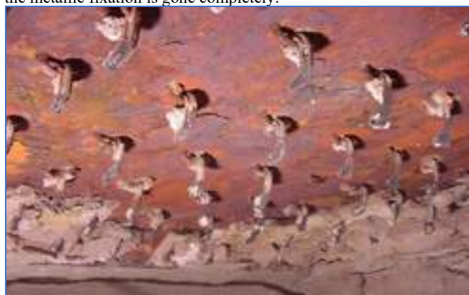
Pic. 1: Corroded anchors, roof section
