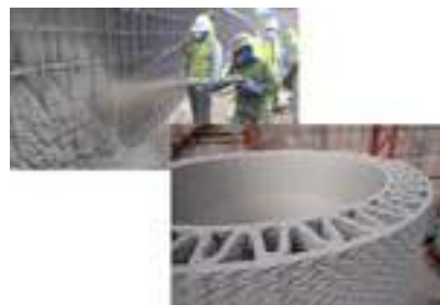
Fig. 5: Examples of shotcrete and novel installation geometries.
