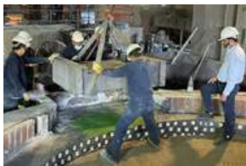
Fig. 4. Setting in place the preassembled slag door block.
