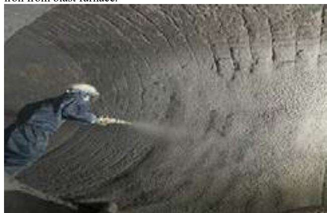
Fig. 1. Shotcrete repair in torpedo ladle car
