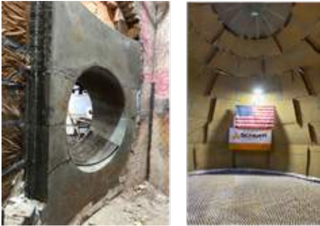
Fig. 6: Burner inlet pour (left) and complete castable dome (right).
