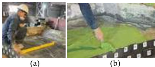
Fig. 3 (a) check the flatness, (b) mortar patching.
