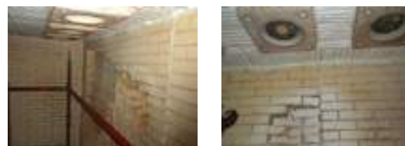
Fig. 3: Deteriorated refractory around burners.
