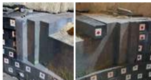
Fig. 5. after setting the upper shell (a) left and (b) right pillar bricks were set as connection to the wall lining.
