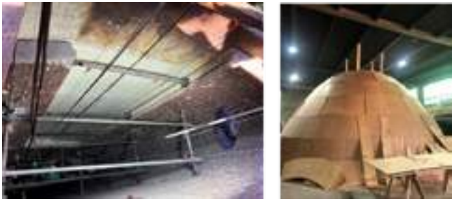
Fig. 5: Bracing the existing walls during demolition (left) and fabrication of the dome forms (right).
