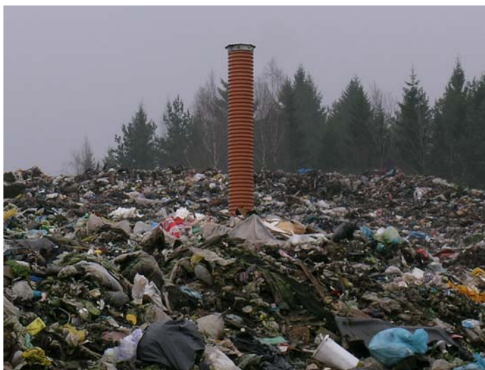
Fig 2.4. Monitoring well (Gas. No. 1) in Jerubaiciai landfill cell No 1.
