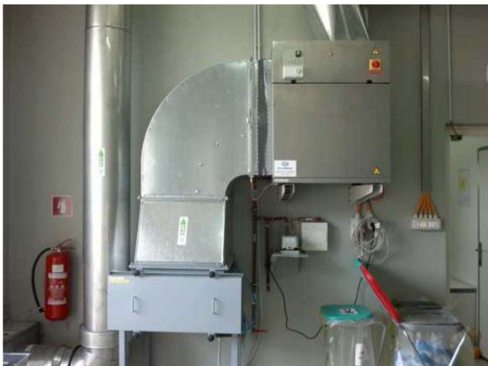
FIG. I–13. Heating and moisture control system.
