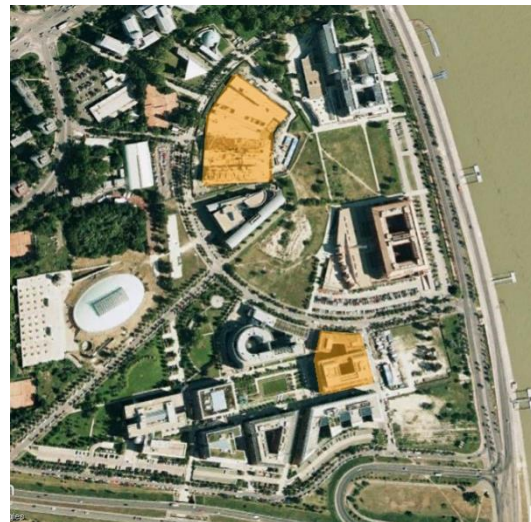
Fig.3. Pilot area in September 2009 (Orange buildings were built in the 3. period)
