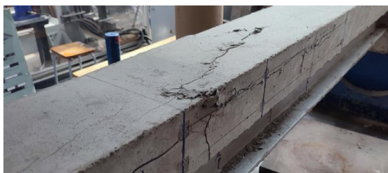
Fig. 3.21. Hybrid beam failure because of the concrete crushing (made by the author)
