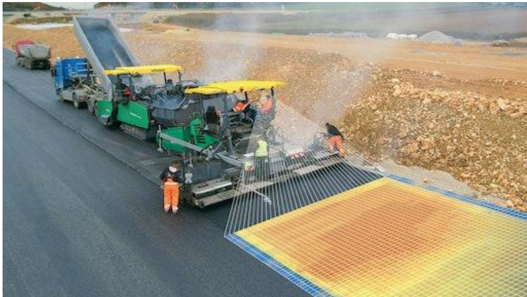
Fig. 21. Temperature registration behind the paver with thermal camera
