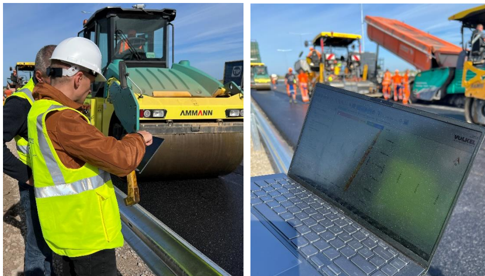
Fig. 31. Temperature registration after each pass of the roller through a specific point
