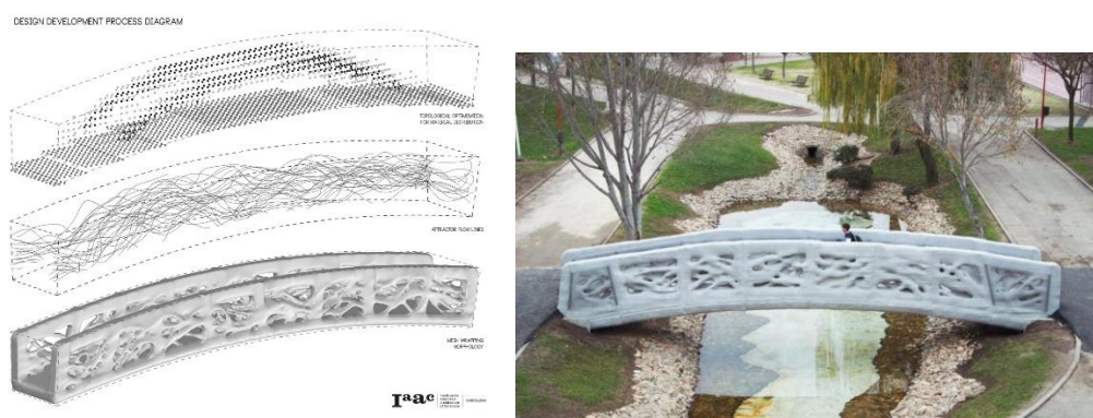
Fig. 1.5. Castilla-La Mancha 3D bridge (Buchanan & Gardner., 2021).
