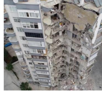
d) Torsional irregularity (Adana)
