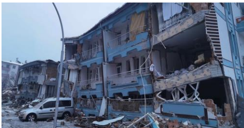
a) Soft storey irregularity-Column rupture (Kahramanmaraş)
