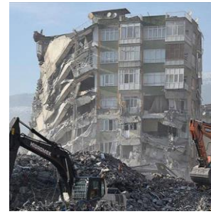
c) Torsional and soft storey irregularities (Gaziantep)
