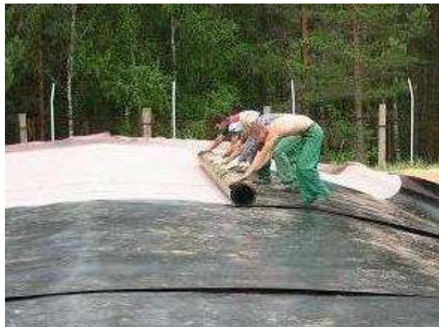
FIG. 4. Installation of HDPE at the facility in 2006.
