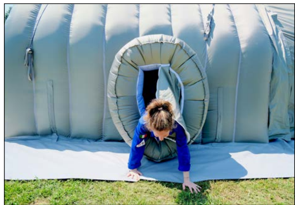
Fig. 10. Simulated porthole in the inflatable structure of the ESH-X habitat.
