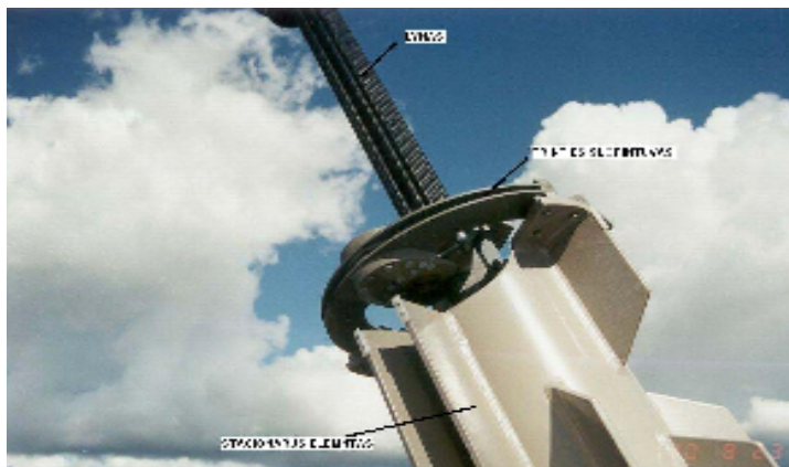
4.25 pav. Trinties slopintuvai vantui [12]
