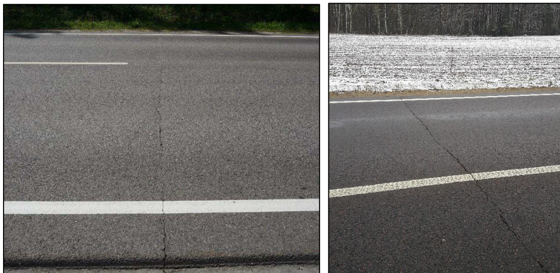
Figure 3: Low temperature cracking
