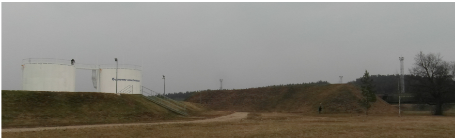
Fig. 3.14. Two views of the soil embankment built in the Lithuanian railway infrastructure to protect fuel tanks against a potential BLEVE on tracks (the top photo was obtained from maps.lt website, the bottom photo was made by the author)
