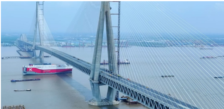
Fig. 1.4. Changtai Yangtze River Bridge (Yang, 2025)
