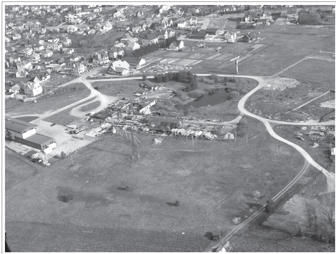
Fig. 2. The obstructed Karmėlava ancient cemetery: the view from the west (25 April 2007) (photograph by G. Zabiela).
