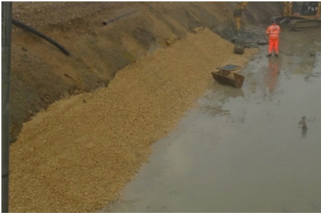
Figure 7 Construction of Angular Drainage Stone Key
