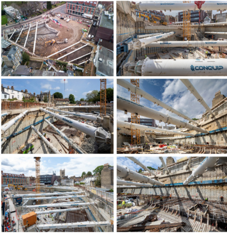
Figure 7 Basement Excavation & Propping
