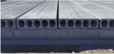
Figure 5 Precast hollow-core foundation slabs
