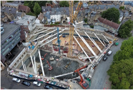
Figure 1 Basement Excavation and Propping
