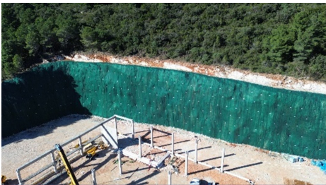
Figure 4 Finished part of the protected slope
