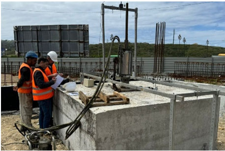
Figure 6 Full scale tension load test
