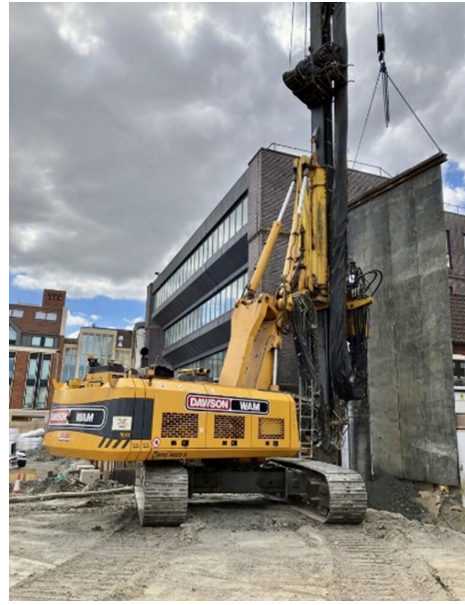
Figure 5 Close Proximity Piling
