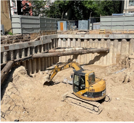
Figure 2 Construction site and retaining walls
