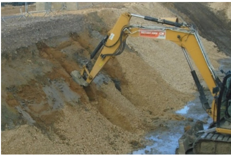
Figure 8 Construction of Cemented Aggregate Columns
