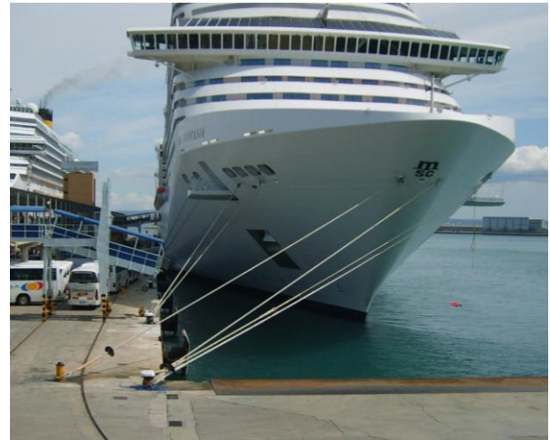
Fig. 13 Possible additional storm bollards on quay the wall for increasing its mooring possibilities
