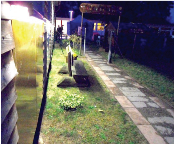
LED-lines for path lighting, RZB, 4 x 9 W, 3.300° K.
