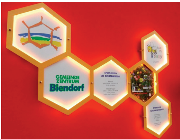
Flexible LED-lines for backlighting the name boards of the kindergarten, Osram, 80 W, 3.300° K.
