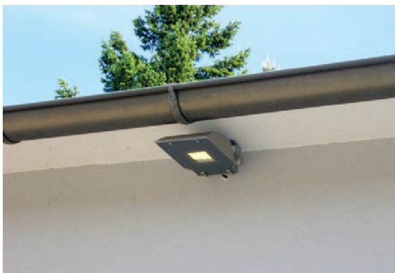
Sill LED spots for lighting up parking ground and entrance 8 x 30 W, 3.300° K, dimmable.
