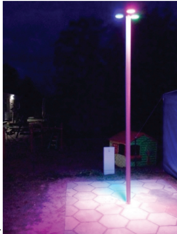
Children's game with colour mixing – Sill RGB-spots with light control for colour mixing, 3 x 80 W.
