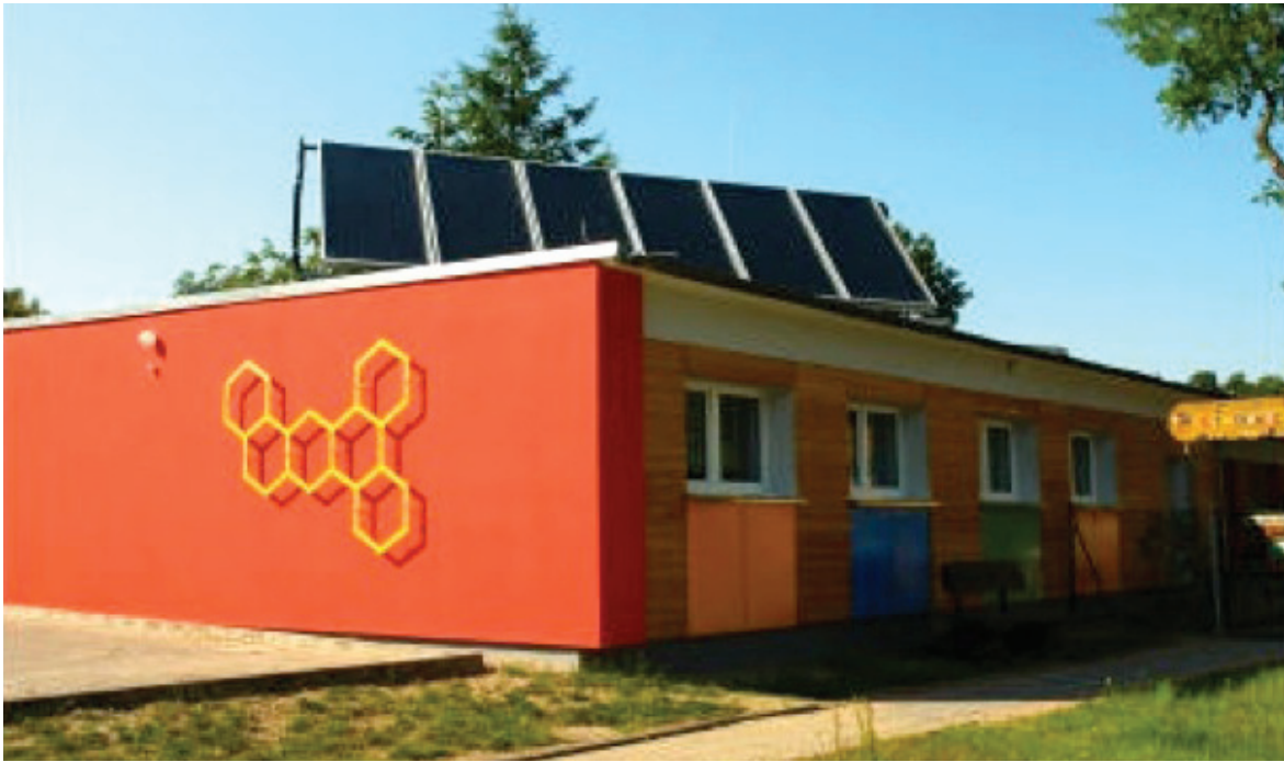
Test area kindergarten and community centre
