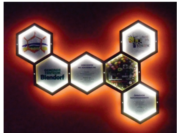
Flexible LED-lines for backlighting the name boards of the kindergarten, Osram, 80 W, 3.300° K.
