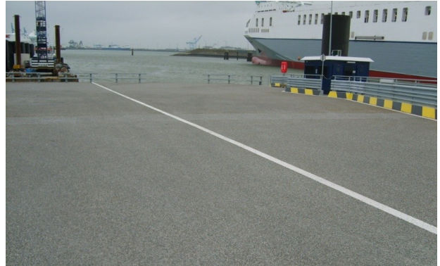
Fig. 7. Pontoon ramp with two loading lines
