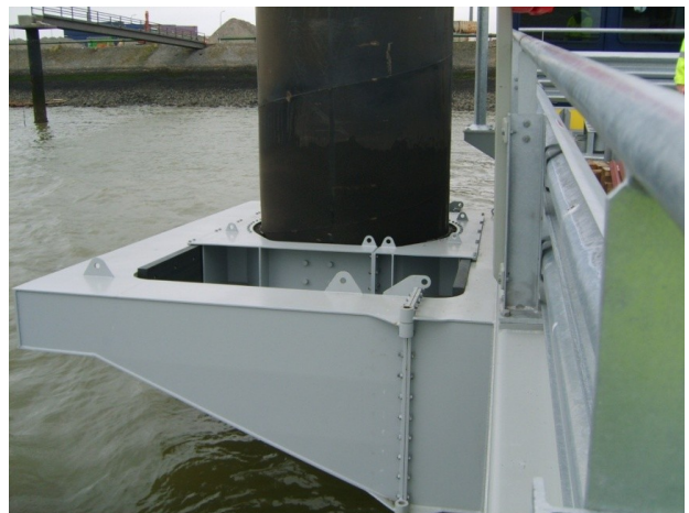
Fig. 8. Pontoon ramp pile anchor with possible ramp movement
