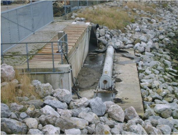
Fig. 5. Link point of the pontoon
