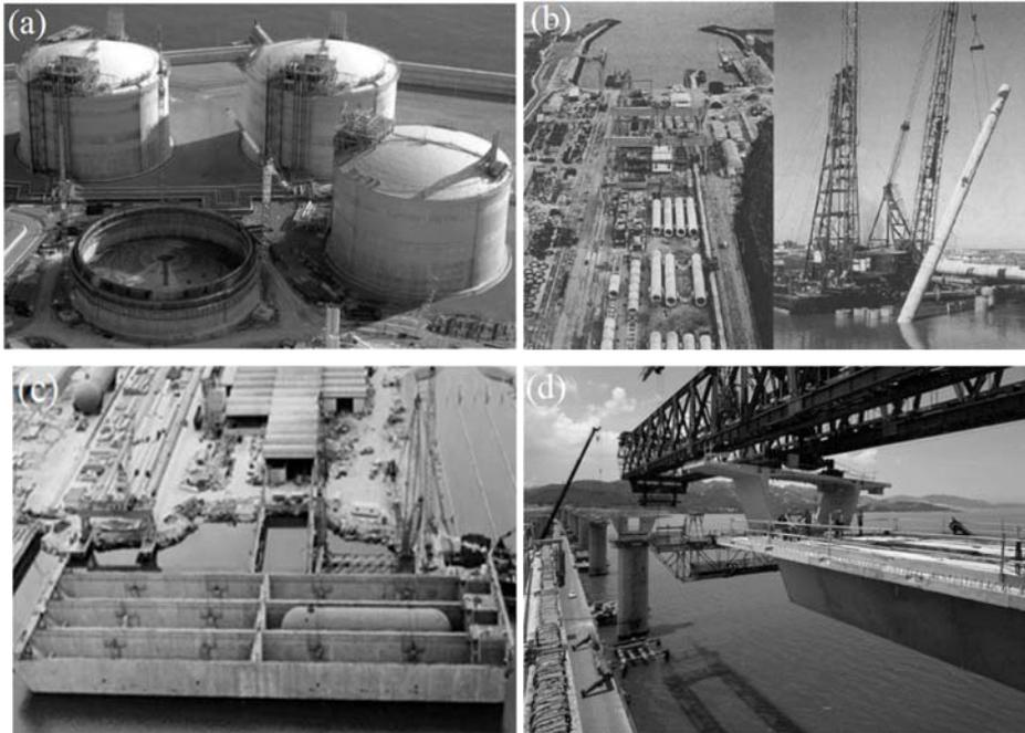
**Fig. 1.1.** Potential employment of prestressed concrete for: liquid storage tanks (Ghali 2017) (a); port deep piles (Tsinker 1997) (b); floating barge units (Gerwick 1992) (c); long-span bridges (Bhatt 2011) (d)
