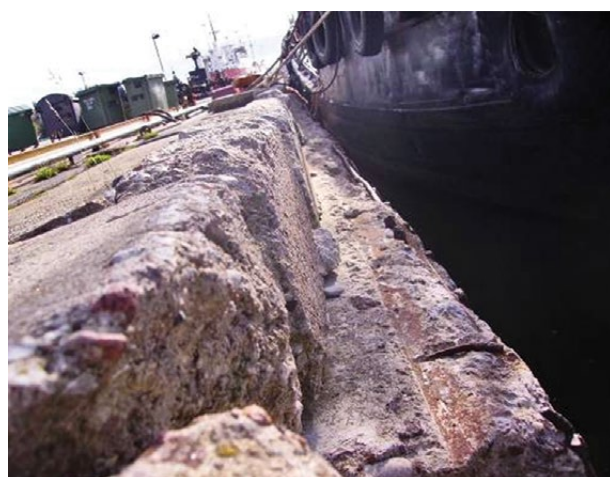
Fig. 9. Mechanical damage to the quay at the Port of Klaipėda
