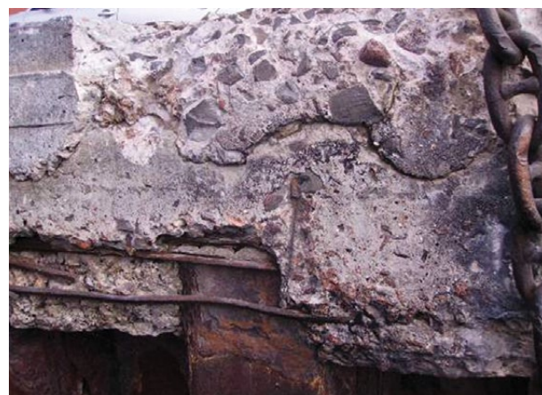
Fig. 8. Mechanical damage to the quay at the Port of Klaipėda
