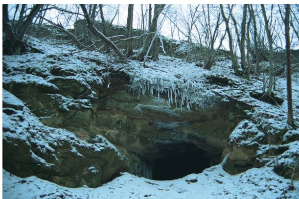
Figure 2. Main entrance of the underground tunnel where observations were made in January and February 2006 (January 2004; photo by Matti Masing).
