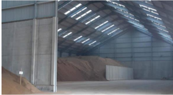
Fig. 11 An internal mobile wall inside a sector
