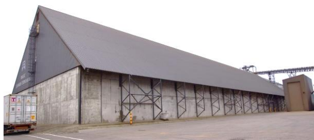
Fig 4 An outside view of the storage facility
