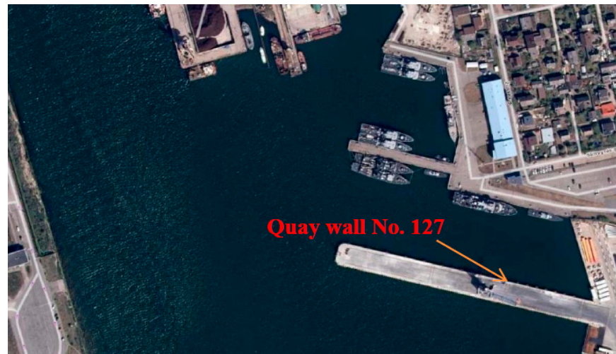
Figure 7. Navigational conditions at quay wall No. 127 area.
