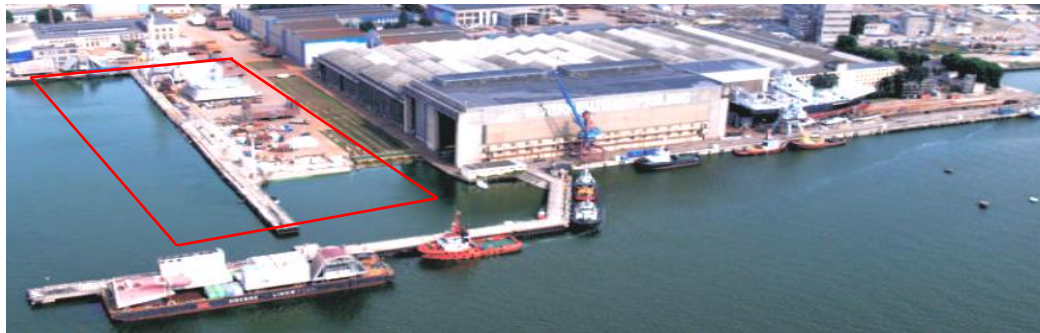
Fig. 1 A general view on the seaport shipbuilding (with the marked open site) in Klaipėda, Lithuania, the EU
